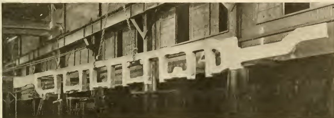
VANADIUM CAST STEEL FRAME FOR NEW YORK, ONTARIO & WESTERN, 2-10-3 TYPE LOCOMOTIVE Union Steel Casting Co., Makers.
